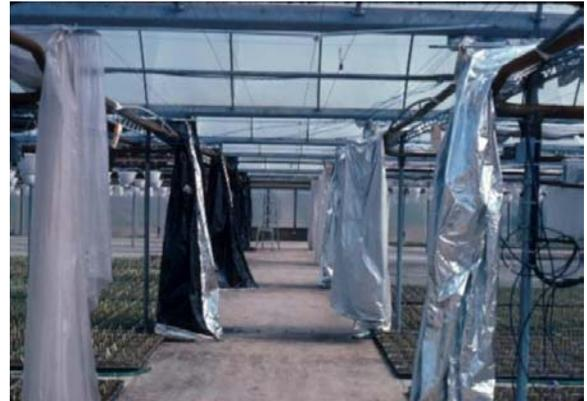
The curtains drawn from gutter to gutter in this installation with tails to seal at the gutters provide an insulated attic space under the double-poly roof (left). With 10 bays and 20 sections to curtain off there was the opportunity to evaluate a variety of potential materials (right). The curtain closing over an early fall poinsettia crop is shown below.
