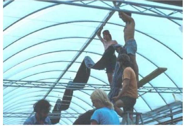
Installation of test curtain materials in 0.54-hectare greenhouse before the development of modern curtain pulling systems was a challenge. The students figured out a pulley system to draw the curtain over the galvanized trusses without tearing the material.
