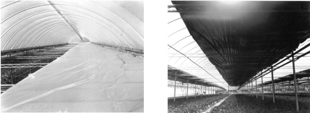
Fig. 6 Curtain System Viewed from Above and Below while Closing
