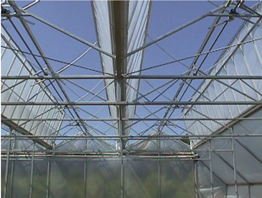
View showing the clear sky through the roof on June 11, 1999
