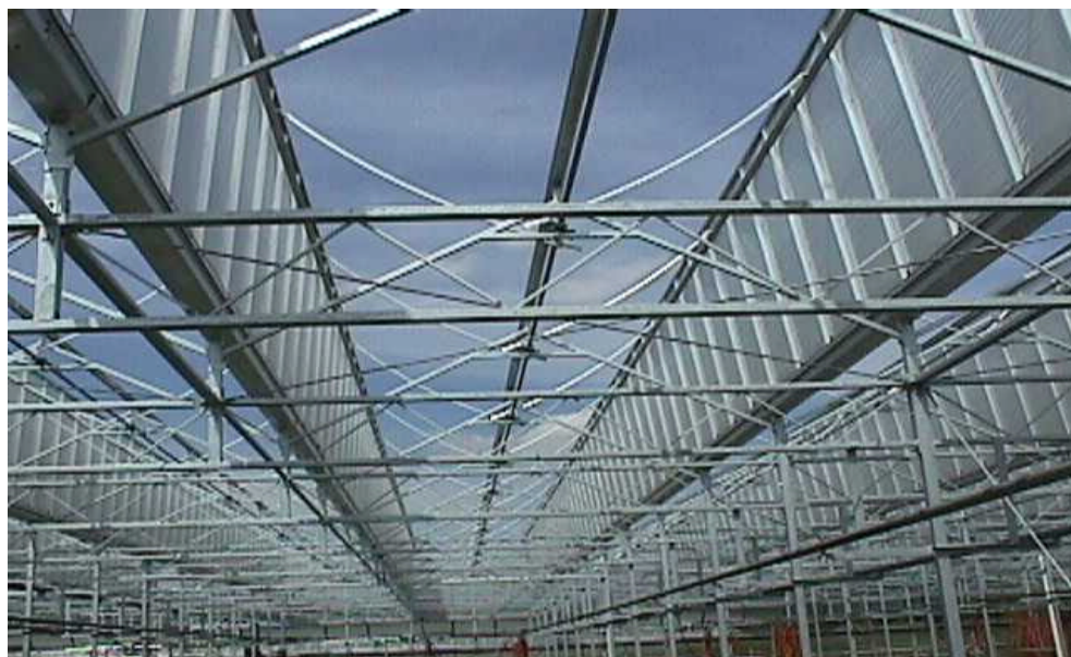
Ken Van Wingerden's open roof, double poly glazed greenhouse, Pompton Plains NJ 9/3/98
