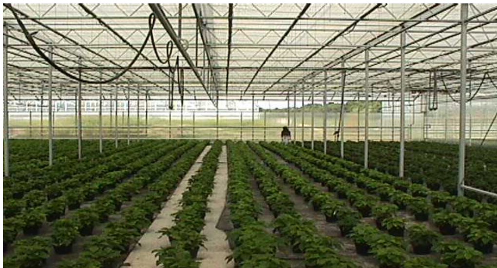
Neil De Groot's conventional double poly greenhouse with thermal screen in position. 9/3/98
