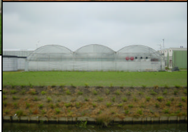
The first air-inflated-double-layer polyethylene greenhouse in the world 2003.
