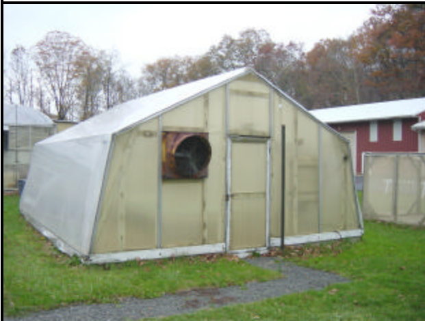
The first air-inflated-double-layer polyethylene greenhouse in the world 2003.
