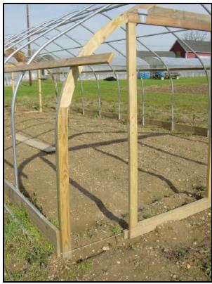
The bottom of the large hinged door extends a little into the soil to create a sill-less entry for soil tillage equipment. To open the door, some soil will have to be removed.
