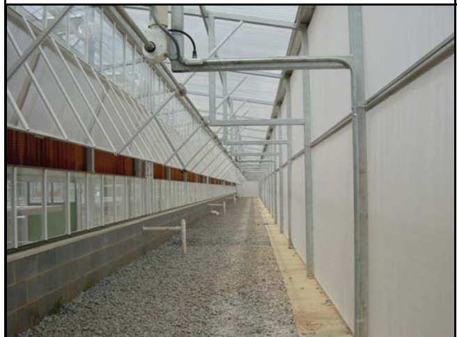
Photo 2. NSCU, inside the screening enclosure with the insect screen on the right and the ventilation inlet opening on the left (with evaporative cooling pad).
