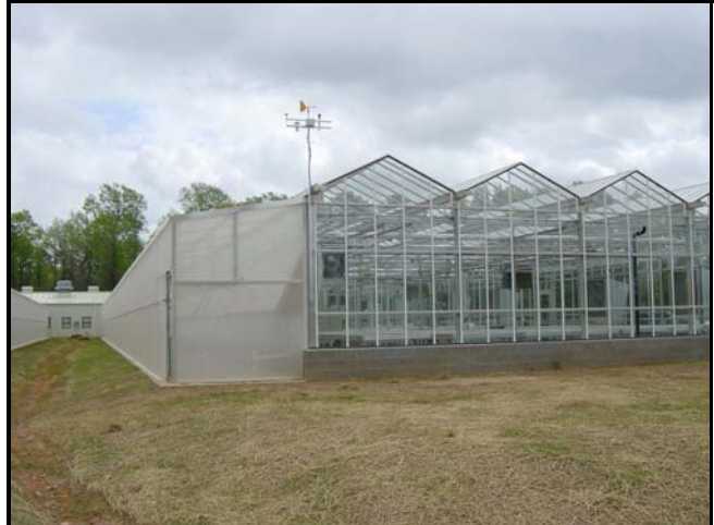
Photo 1. NCSU, the new teaching and research greenhouses with insect screening. An enclosure was constructed along the sidewall with the ventilation inlet opening.
