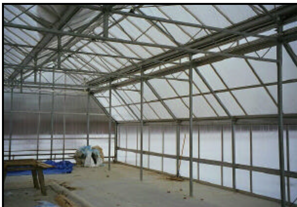
Interior view of the open-roof greenhouse. The sidewalls are twin-walled acrylic panels (16 mm thick), the roof segments are double poly. Note the snow on the roof near the gutter.
