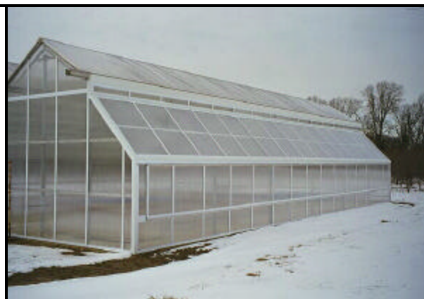
Exterior view of the open-roof greenhouse (East wall). The vertical portion of the East wall was outfitted with a continuous side vent. A similar vent was installed in the West wall.
