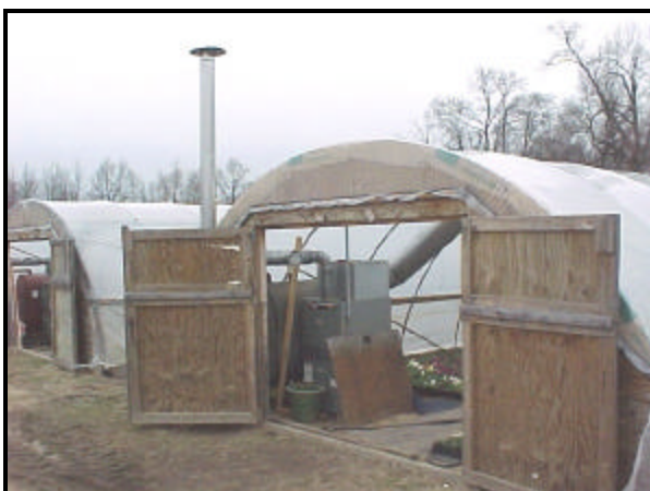
Greenhouse heating system.
