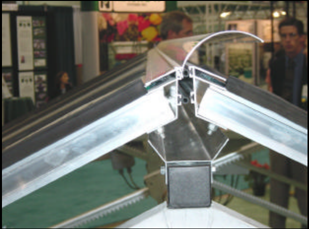
Design detail of the peak of an open-roof greenhouse.
