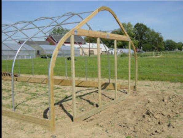
One of the frames of the large hinged end wall doors is installed. These doors (at both ends) allow for a small tractor to drive through the tunnels while preparing the soil and making the raised beds. Note that the door extends beyond the surface of the soil. Therefore, the doorframe is made of pressure treated wood and some soil will have to be removed when the doors need to open for the infrequent soil preparation with the tractor.
