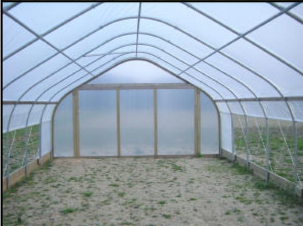
Inside view of the high tunnel structure. The soil will be tilled and the four slightly raised beds will be covered with a black plastic mulch. The plants will be irrigated using drip tape. A fertilizer injector will be used to provide the plants with the required nutrients. For more information on crop production in high tunnels, please visit the following web site:
