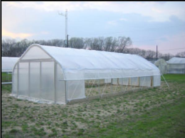
Finished structure of one of the high tunnels. A single layer of 6 mil polyethylene (4-year film) covers the entire structure. Roll-up side walls can be raised and lowered depending on the need for ventilation. A lattice of rope prevents the roll-up sides from damage due to high winds. A single person entry door (not visible) allows access throughout the growing season. Two of the high tunnels are outfitted with thermostatically controlled roll-up sides (requiring electric motors).
