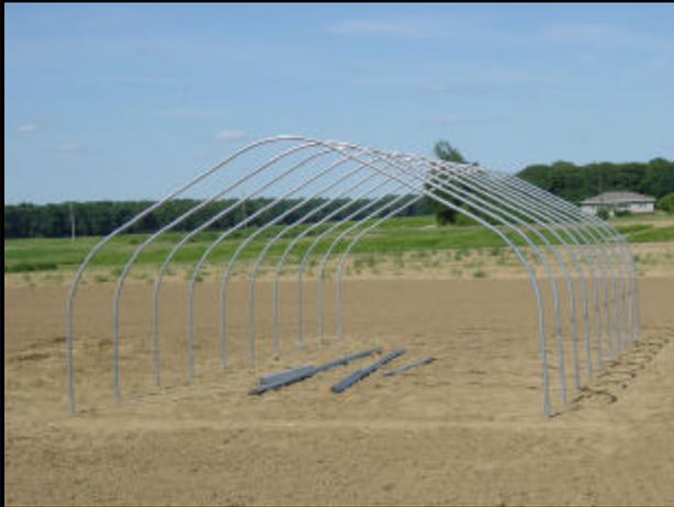
A total of 10 bows for a 17 by 36 feet high tunnel are installed. Cross braces will be installed to give the structure extra strength. Such high tunnels are mainly intended as season extenders: because the plastic covered structure and the plastic mulch can protect a crop (to a certain degree) from adverse weather conditions (especially cold temperatures), a grower is able to start earlier and continue longer in the season. Hopefully, a better market price will offset the cost of the structure.
