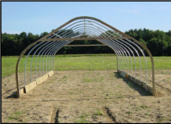
Pressure treated sideboards are installed along the sidewalls of the high tunnel.
