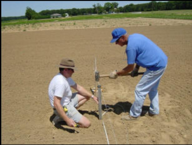
The high tunnels measure 17 feet wide by 36 feet long. The position of each foundation posts is carefully marked by strings, and the distance between the posts is 4 feet. The foundation posts are hammered into the ground. A large bolt is temporarily placed on top of the hollow post to protect it from deformation during placement. Four high tunnels are installed at the Rutgers Agricultural Research and Extension Center (South Jersey) and two at the vegetable research farm on Cook Campus.
