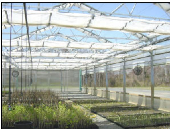
Retractable Roof Greenhouse with Shade Curtain
