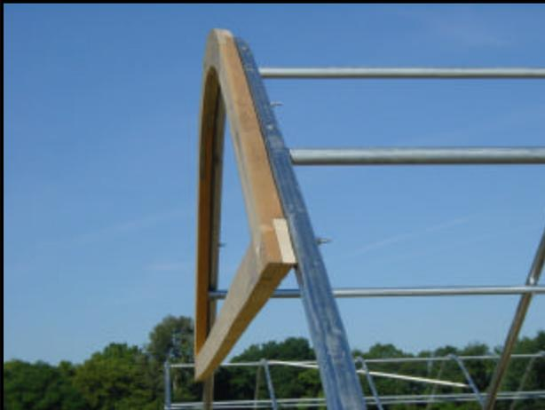
Wood pieces are bolted to the end wall bow to allow for a place to attach the plastic film. Where the wood starts to curve, two pieces of plywood are lapped and glued together to make for the same thickness as a 2 by 4. All other wood connections are also lapped and glued. This is a little more time consuming, but makes for a stronger and more durable connection. Pressure treated wood is used where the wood is in contact with the soil.
