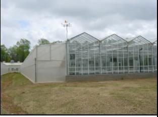
Photo 1. NCSU, the new teaching and esearch greenhouses with insect screening. sidewall with the ventilation inlet opening.
