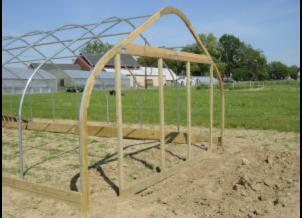
One of the frames of the large hinged end wall doors is installed. These doors (at both ends) allow for a small tractor to drive through the tunnels while preparing the soil and making the raised beds. Note that the door extends beyond the surface of the soil. Therefore, the doorframe is made of pressure treated wood and some soil will have to be removed when the doors need to open for the infrequent soil preparation with the tractor.
