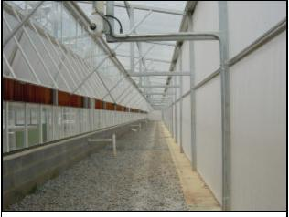
The smaller the screen mesh size, the easier Photo 2. NSCU, inside the screening encloit is for dust particles to collect on the screen sure with the insect screen on the right surface. The dust particles can further reduce and the ventilation inlet opening on the left
