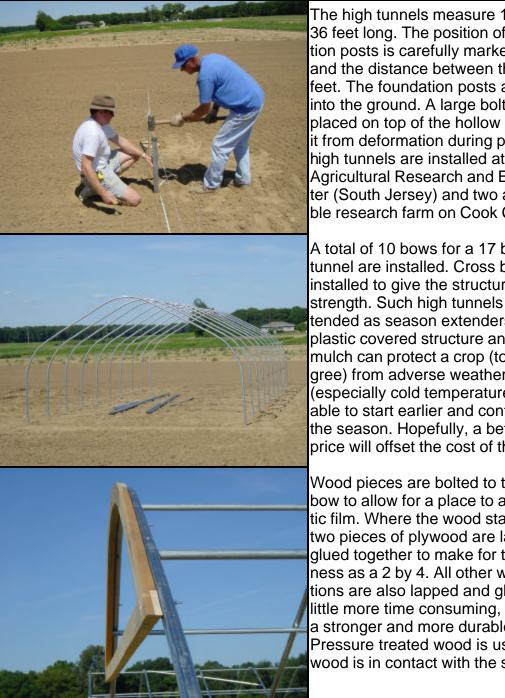
The high tunnels measure 17 feet wide by 36 feet long. The position of each foundation posts is carefully marked by strings, and the distance between the posts is 4 feet. The foundation posts are hammered into the ground. A large bolt is temporarily placed on top of the hollow post to protect it from deformation during placement. Four high tunnels are installed at the Rutgers Agricultural Research and Extension Center (South Jersey) and two at the vegetable research farm on Cook Campus.
