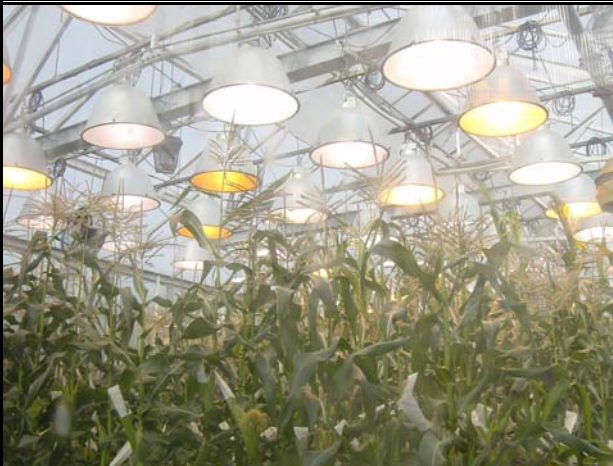
A combination of Metal Halide (white) and High Pressure Sodium (yellow) lamps used to grow an experimental corn crop.
