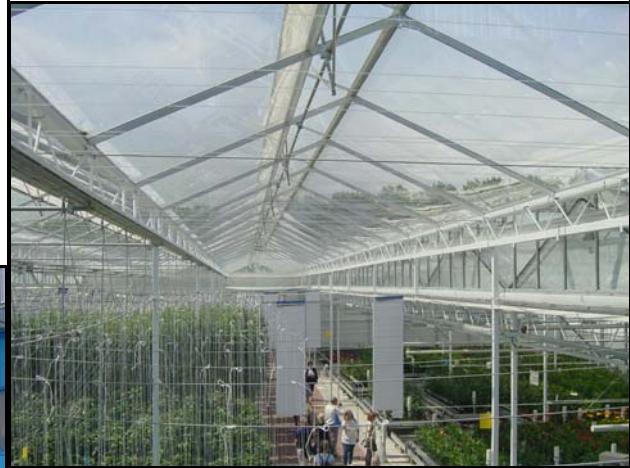
Photo 6. Greenhouse roof construction.
