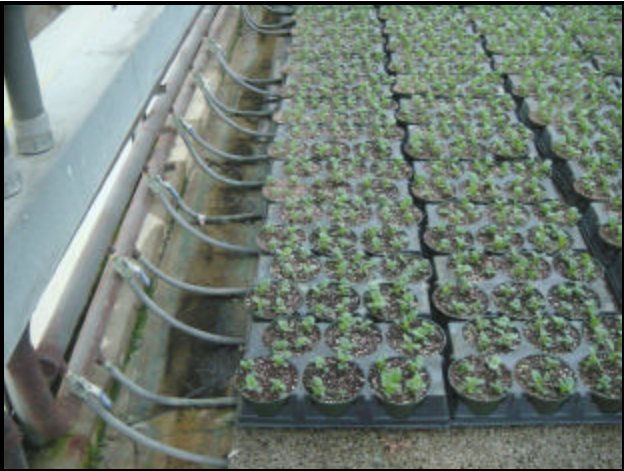
Photo 4. A floor heating system installation using a porous concrete floor (visible at the bottom of this picture).
