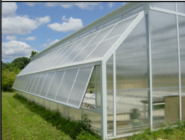
Photo 2. Ventilation inlet opening.
