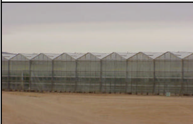
A view of the end wall of the greenhouse.
