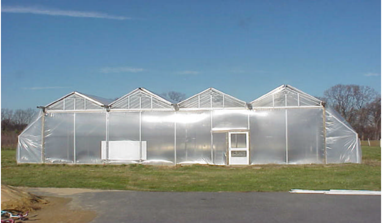
CCEA's open-roof greenhouse research facility located at Rutgers University in New Brunswick, NJ
