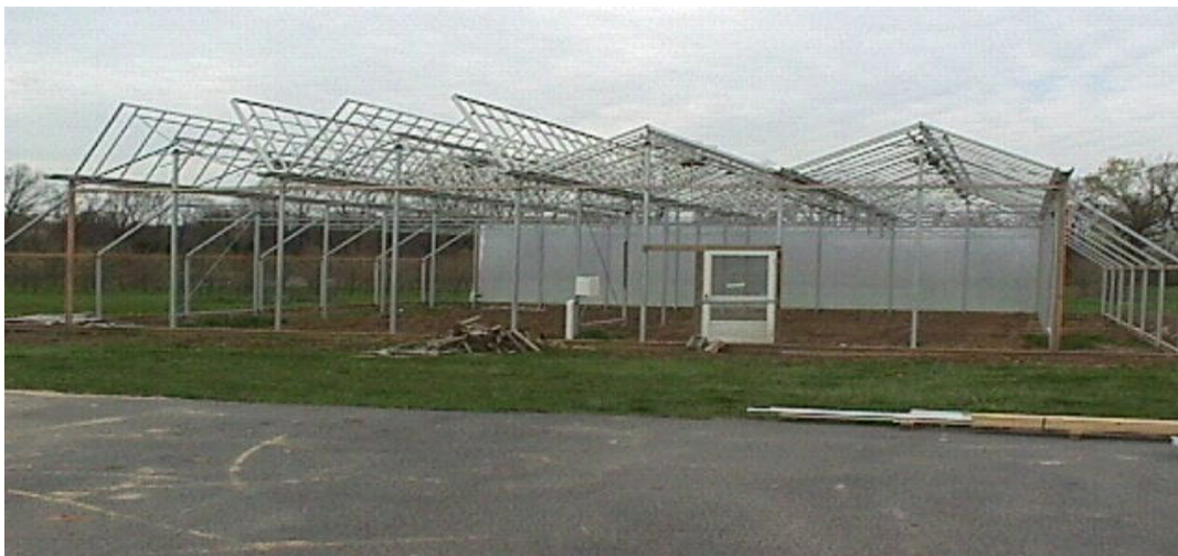
View of Greenhouse during covering in April 1999
