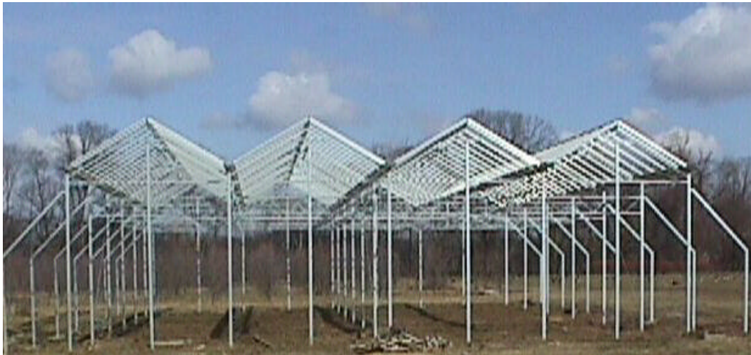
View of MXII greenhouse when superstructure was erected in March 1999
