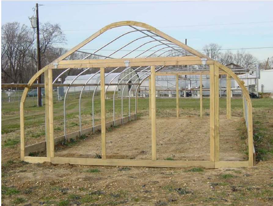
Photo 1. Framed end wall.
