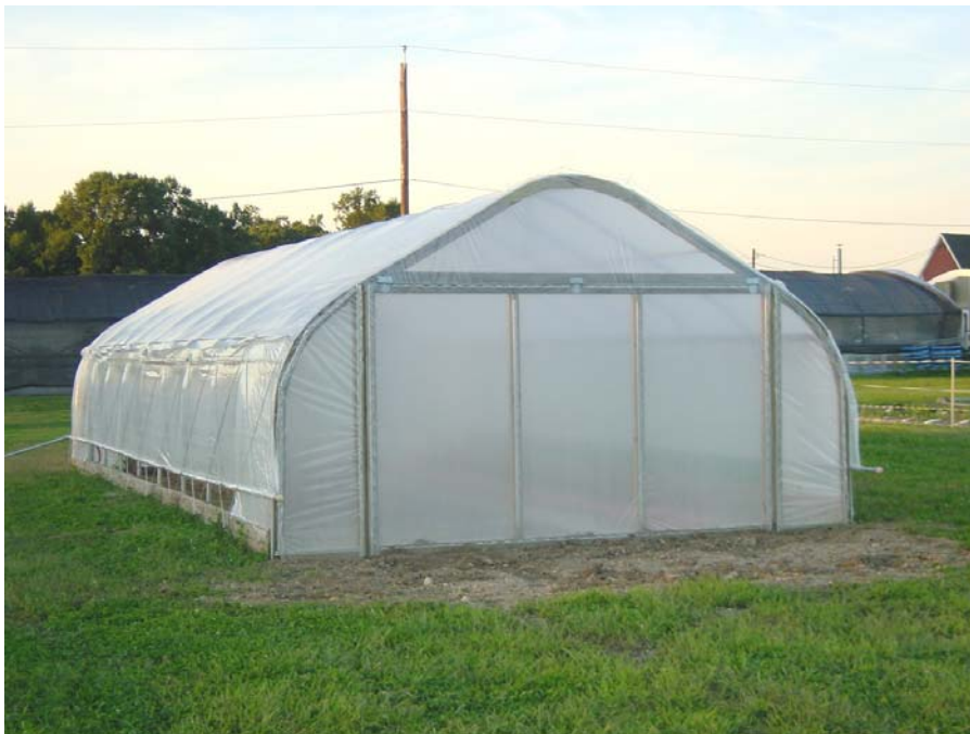
Photo 2. Finished high tunnel with manual roll-up sides.
