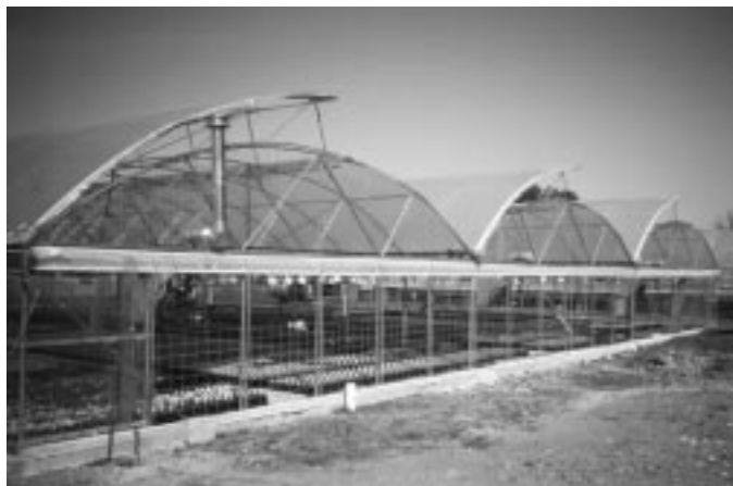
A gutter-connected poly greenhouse with an open-roof design for summer cooling.
